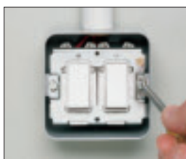
5 Fix wired switch/grid assembly into box.
