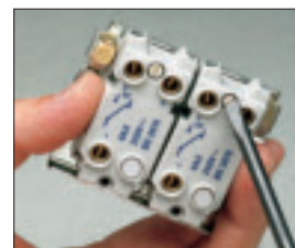
3 Fix switches into grid.
